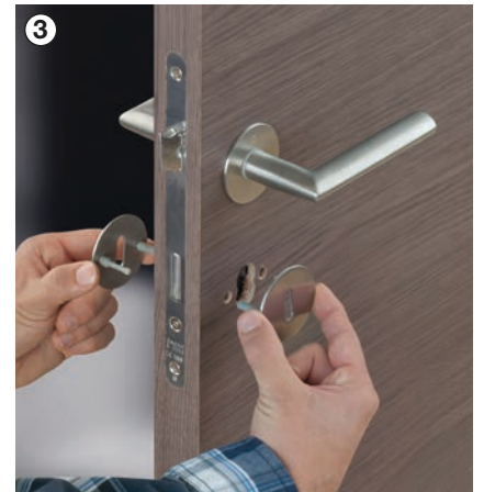
3 Put the escutcheons together – and fitting is complete!
