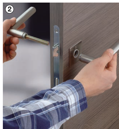
2 Put the door handles together
