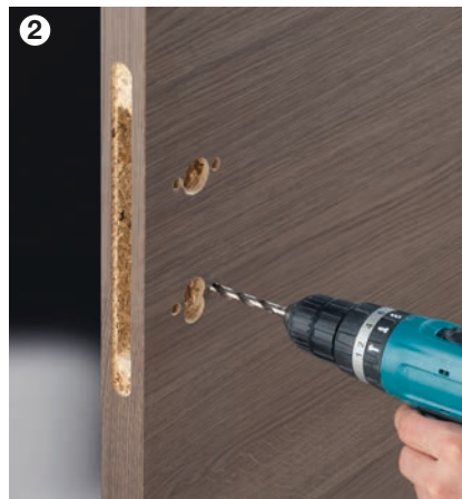
2 Drill the holes for the guiding lugs (remove the lock case for this).
