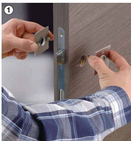
1 Place the handle roses in position
