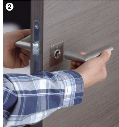
2 Put the door handles together
